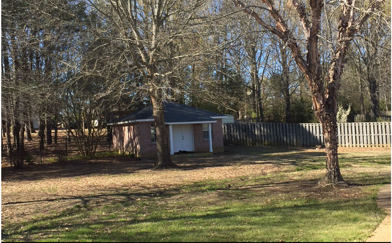
View of existing structure
